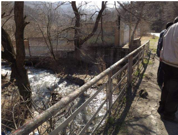
Fig. 8. V. Vahagnadzor, after 30-40 m of nameplate
