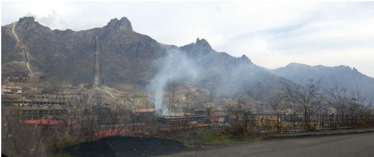
Figure 7 Copper processing plant in Vanadzor
