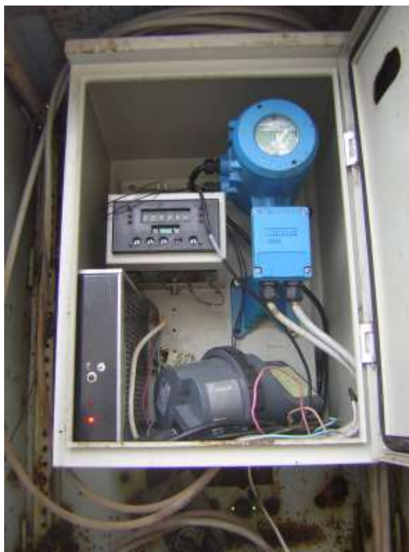
Flowmeter Converter on network with inverter and transmitter of data
