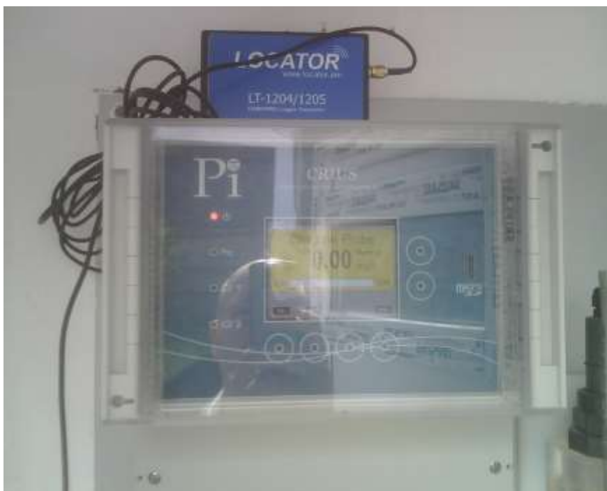
Chlorination Dosimeter with Locator Datalogger
