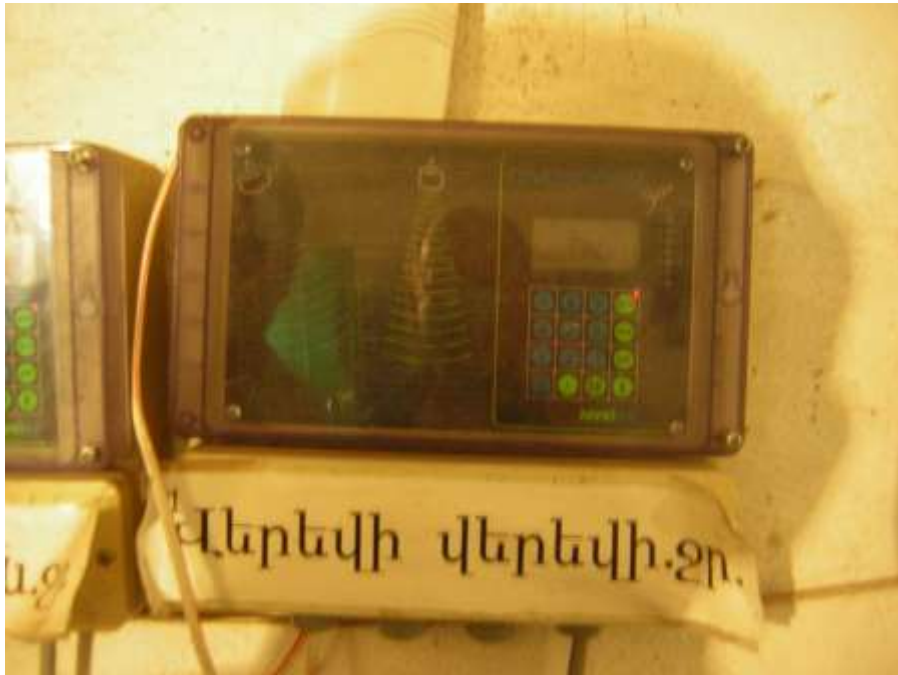
Level indicator in a reservoir.
